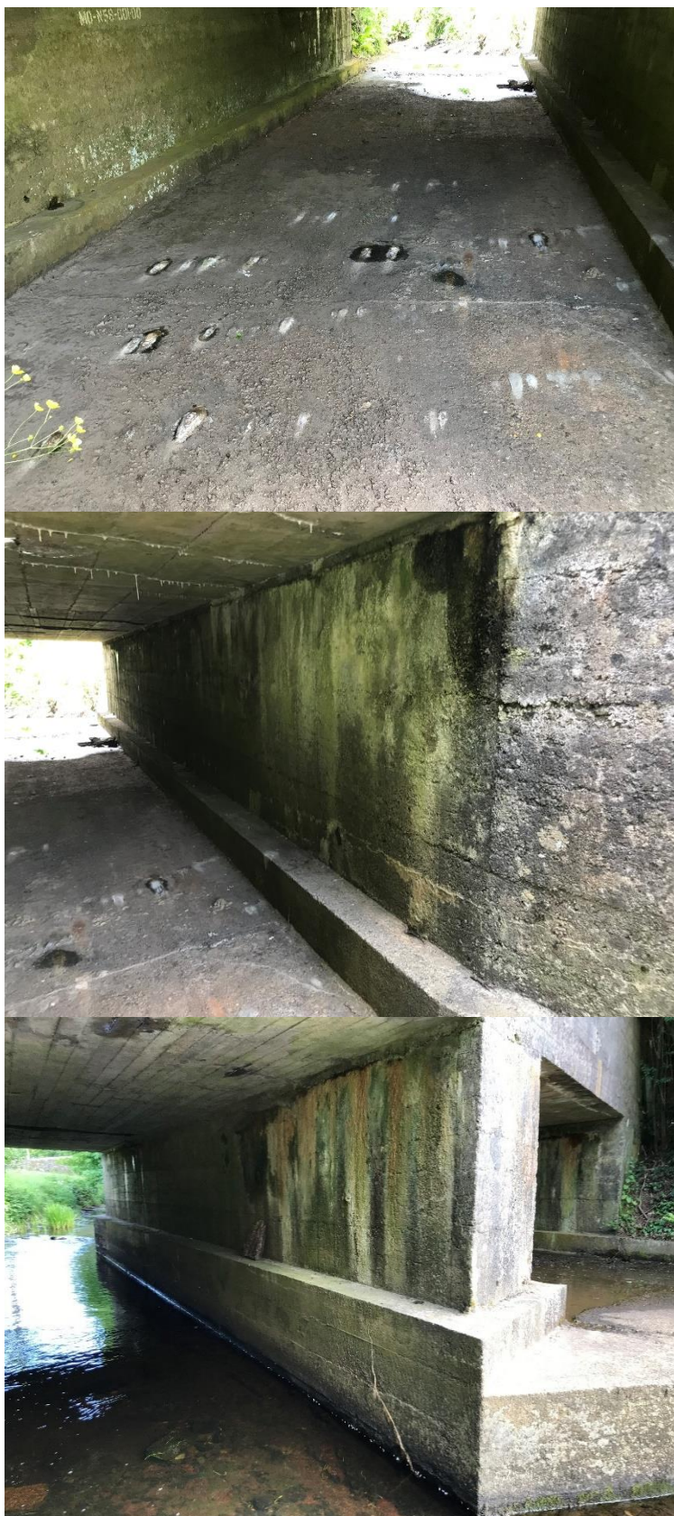
Figure 1-4 – Internal view of the existing concrete apron.
