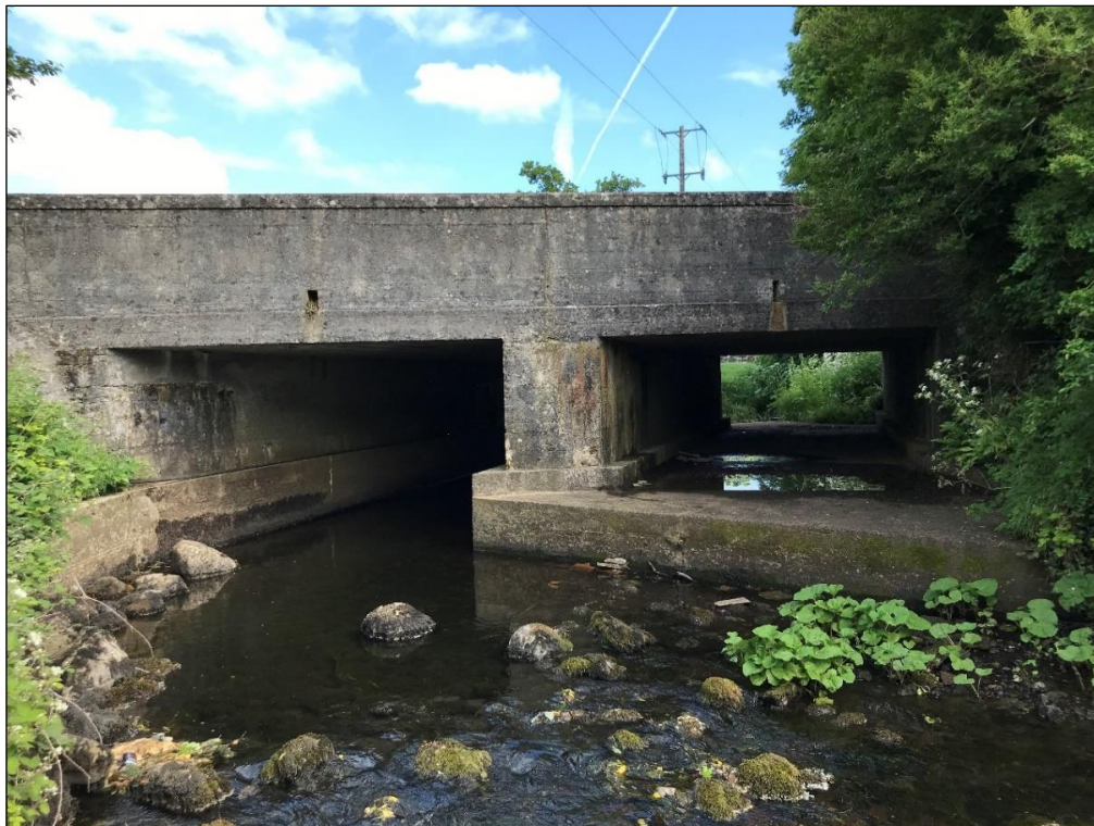
Figure 1-2 – View of the west (downstream) elevation showing the existing concrete apron (on true left bank) with low flow channel in the background.
